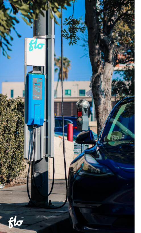
A recent system upgrade saw the department transition to an LED energy system, which resulted in excess available power inside the lighting infrastructure. As part of their commitment to fostering EV adoption inside the city's limits, the city of Los Angeles aspired to using this excess power to install EV charging infrastructure and combat range anxiety.
